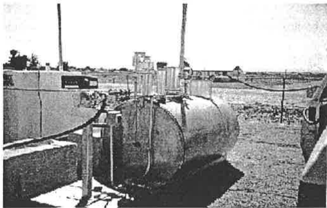
Figure 3. The fuel vault with the blending valve and fuel meter in the foreground and the diesel nurse tank to the left in the background.
